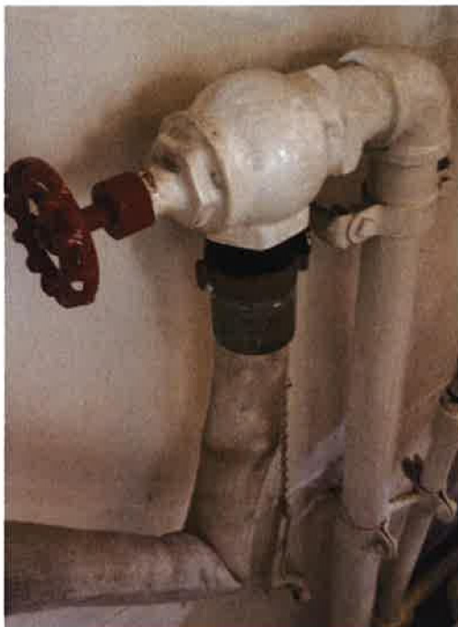
Figure 21-A: Fire Station Valve
