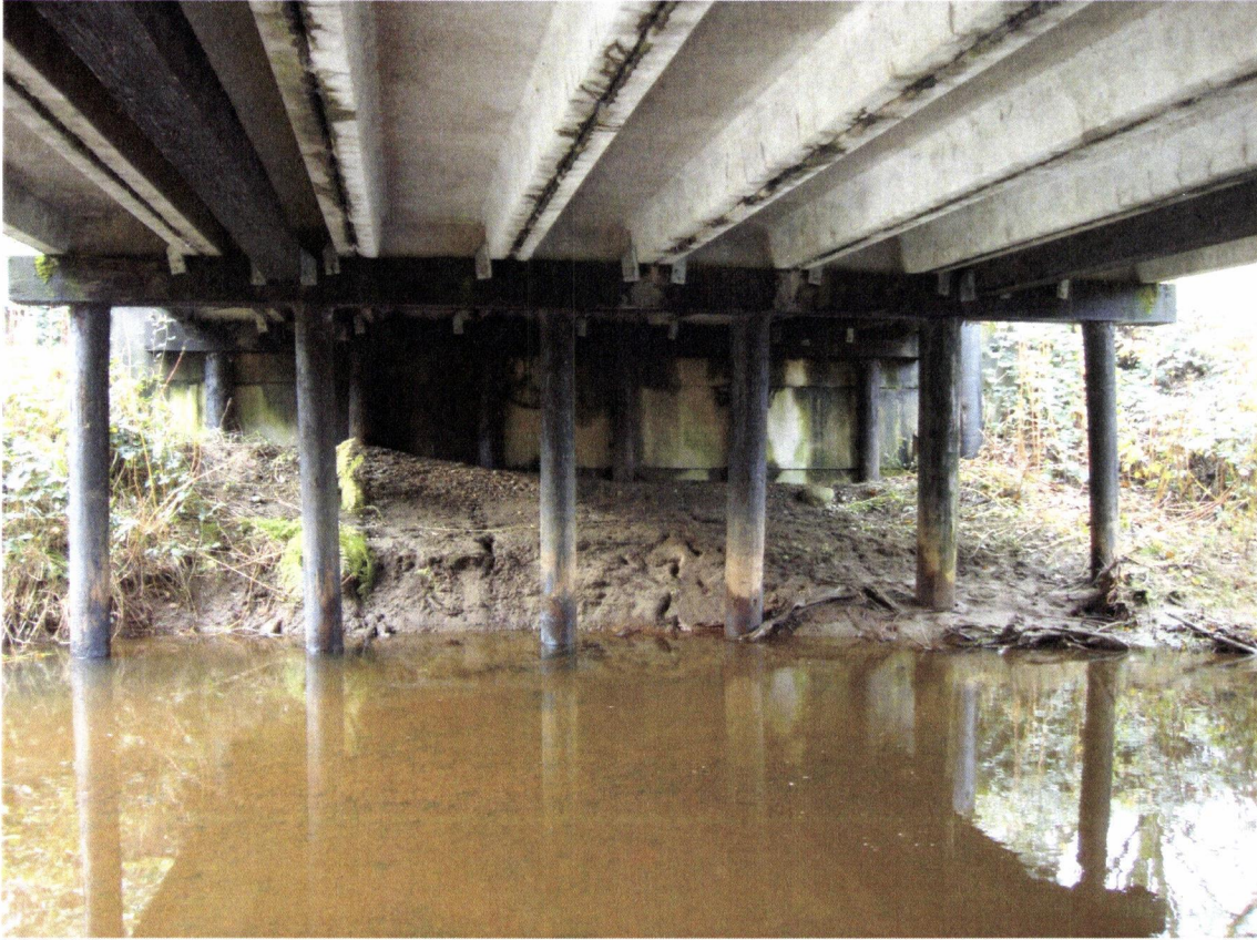
W. Badger Road/Bertrand Creek Bridge No. 50 is typical of our channel beam girders supported by timber piles and caps
