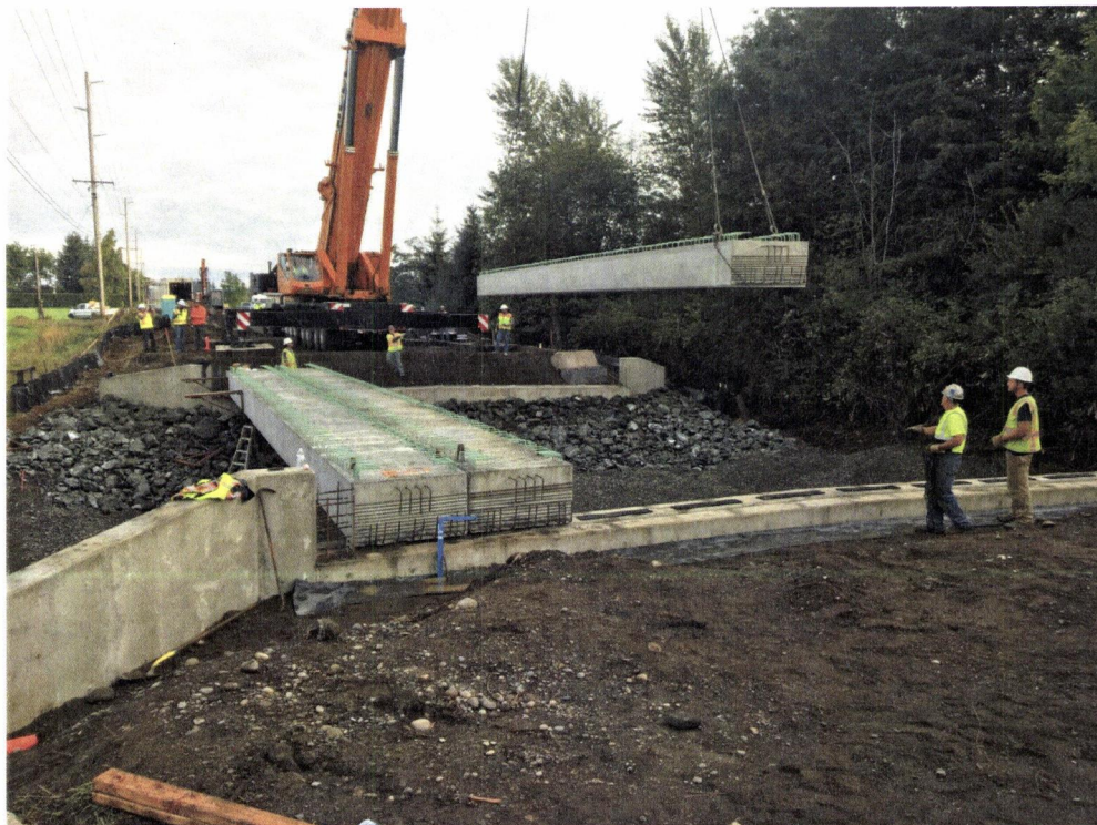
Setting girders during construction of the new Hannegan Road/Ten Mile Creek Bridge No. 236
