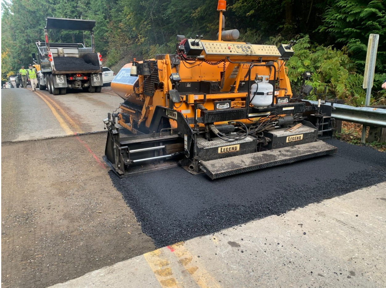
Photo of typical bridge approach repair completed as part of the 2021 Small Area Paving Project.
