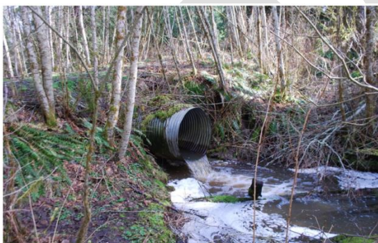
No migration – fish stuck below the culvert
