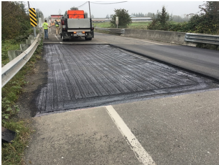
Photo of typical bridge approach repair completed as part of the 2020 Small Area Paving Project.
