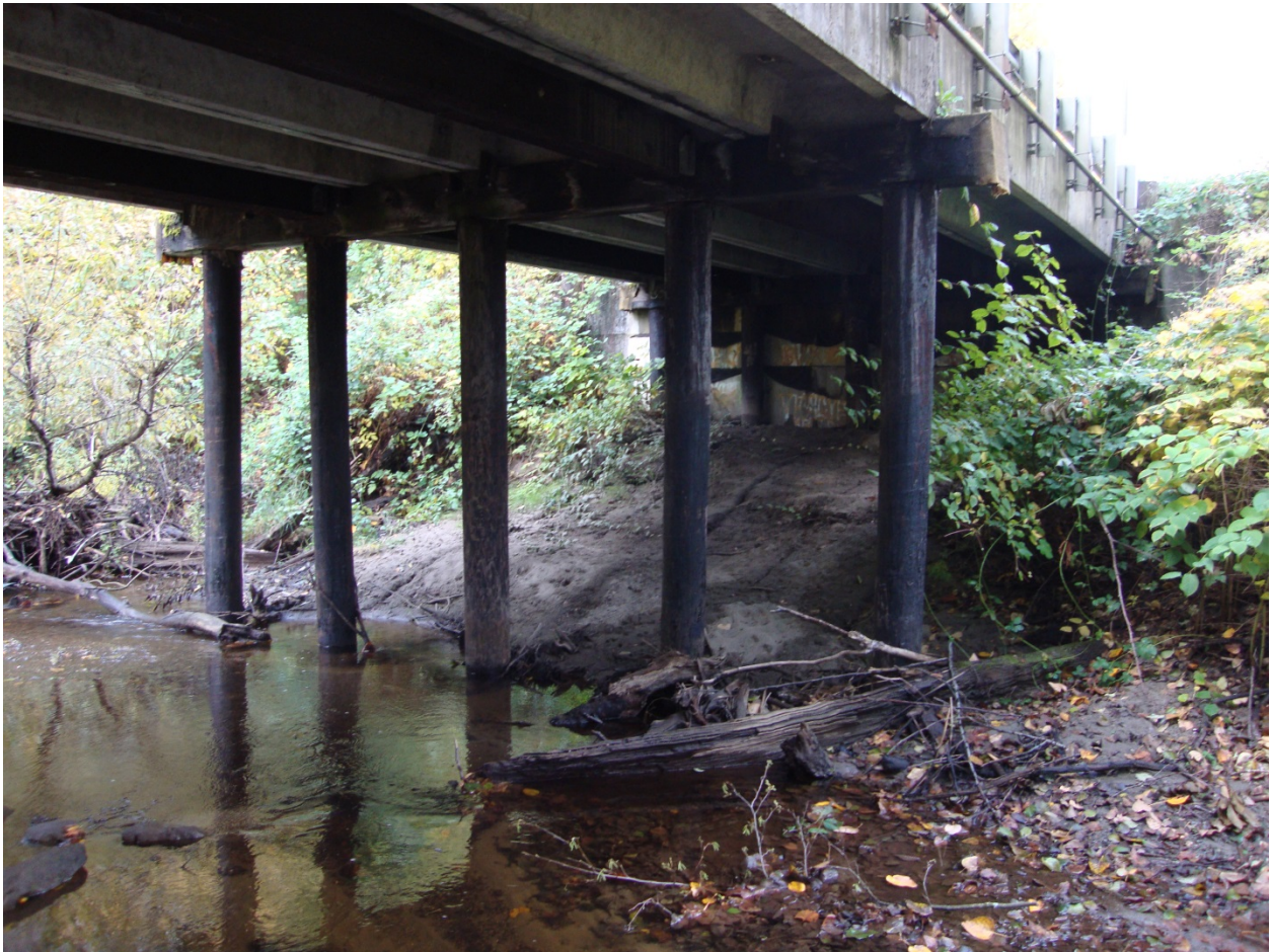
Goshen Road/Anderson Creek Bridge No. 248 is typical of the concrete channel beam girder with timber pile and cap construction which is the most prevalent bridge type in the county inventory.
