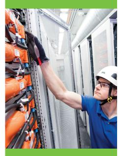
Batteries are placed into removable racks similar to a computer server. There are also monitoring, control and power conversion systems, as well as cooling and fire suppression systems.
