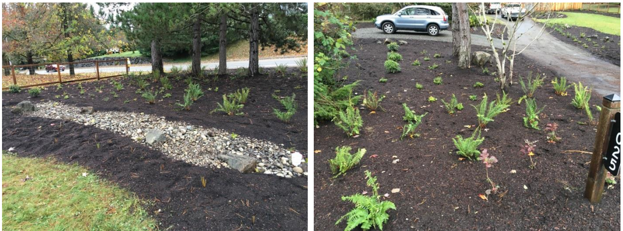
HIP improvements to the McGrath property include large areas of Native Landscaping and a Media Filter Drain treating lawn sheet flow. Total area treated is 18,224 square feet.
