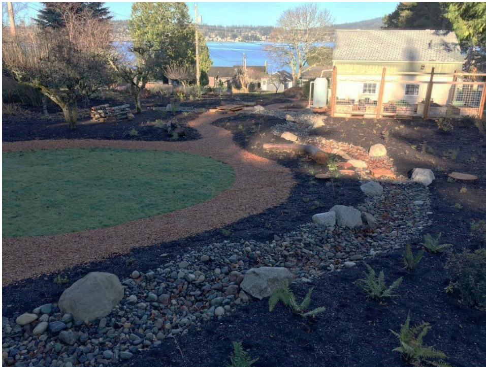
Here is the same large lawn converted to Native Landscaping with a dry creek bed and three dispersion trenches treating a total of 17,410 square feet.
