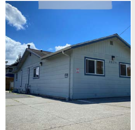
Alabama House 3630 Alabama
