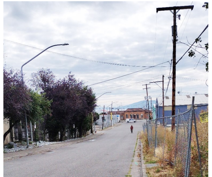
Figure 5. View looking westerly down D Street with the historic BNRR Depot at the terminus. EDI funding would remove utility poles and overhead wires.
