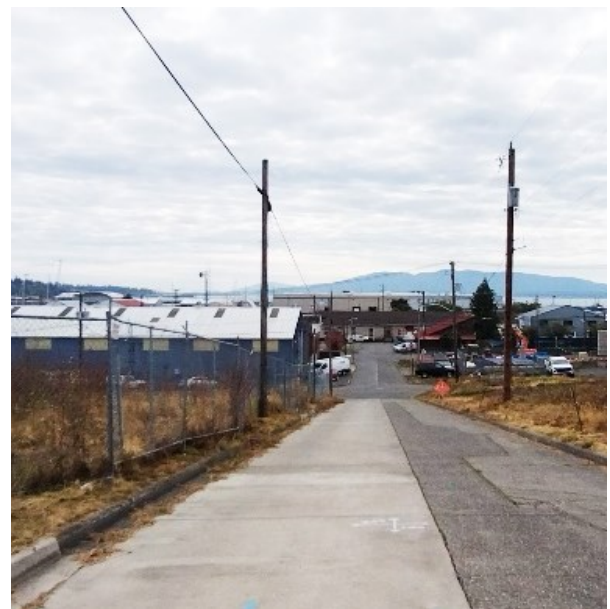
E Street looking westerly. The EDI grant would fund improvements on E Street from Bancroft to Holly Street, underground overhead wires and add intersection lighting.
