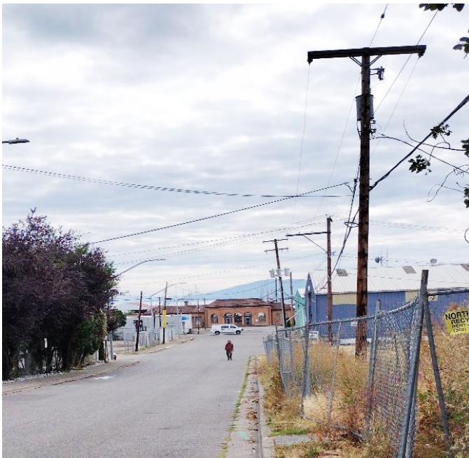
D Street looking westerly. The City will pay for improvements from Holly to Astor Streets – EDI funds would complete the block from Astor to Bancroft, underground overhead wires and add intersection lighting. The removal of distracting overhead wires would enhance the view to the historic BNRR Passenger Station at the D Street terminus.
