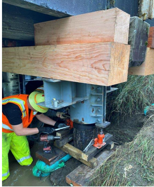
Installation of steel collar brackets on Gillies Road/Sumas River Bridge No. 309.
