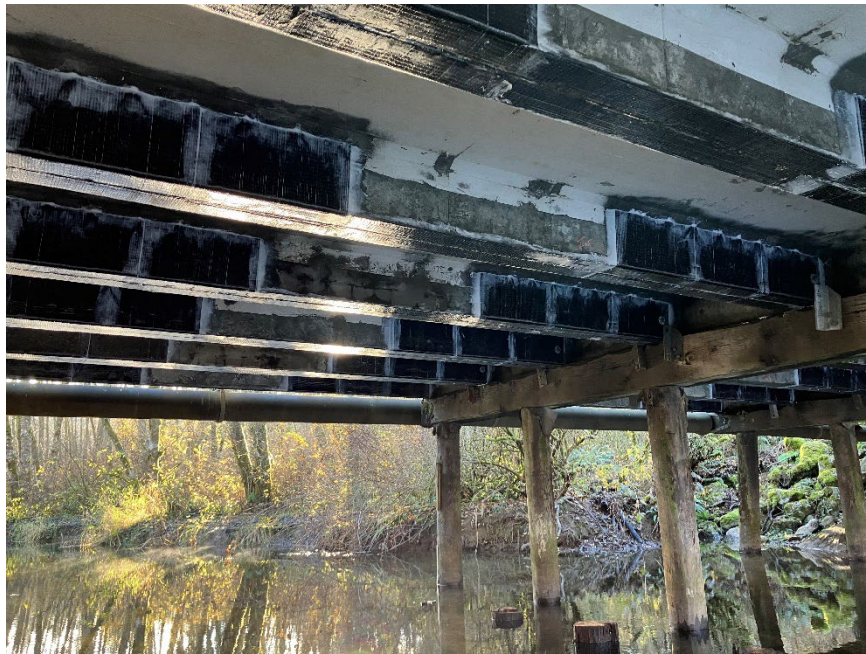
Picture of newly completed carbon fiber reinforced polymer strips to the existing girders on the Nulle Road/Friday Creek Bridge No. 106.
