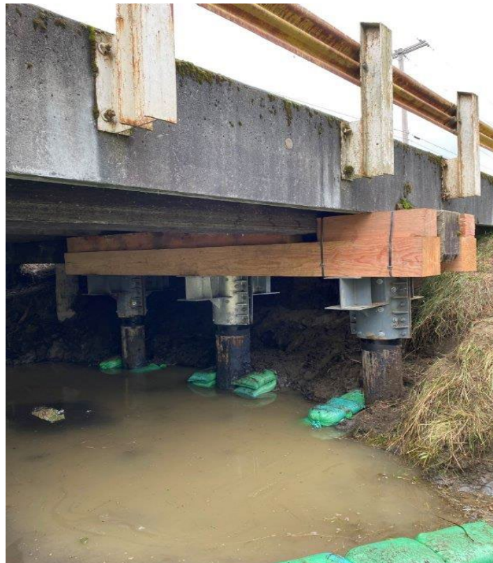
Completed helper timber cap installation at north abutment of Gillies Road/Sumas River Bridge No. 309
