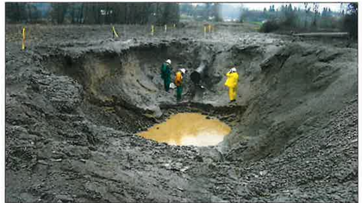
2003 rupture (with no ignition) of a natural gas transmission pipeline near Toledo, WA
