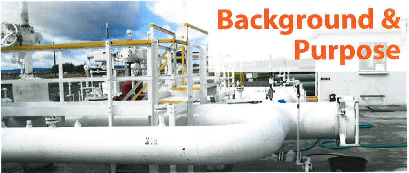
Pig Launchers on a hazardous liquid pipeline near Mt. Vernon, WA
