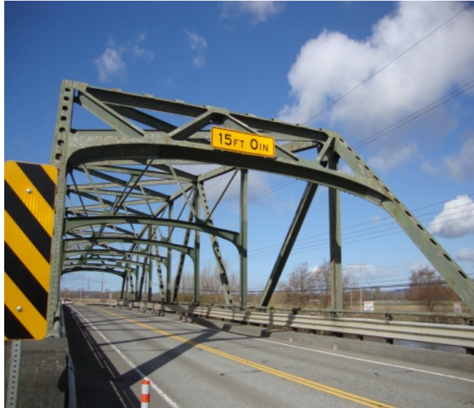
Height restriction sign posted on the Slater Road/Nooksack River Bridge No. 512
