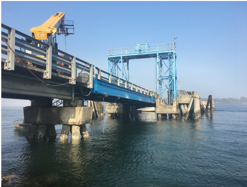
Picture of terminal preservation work at the Lummi Island ferry terminal.
