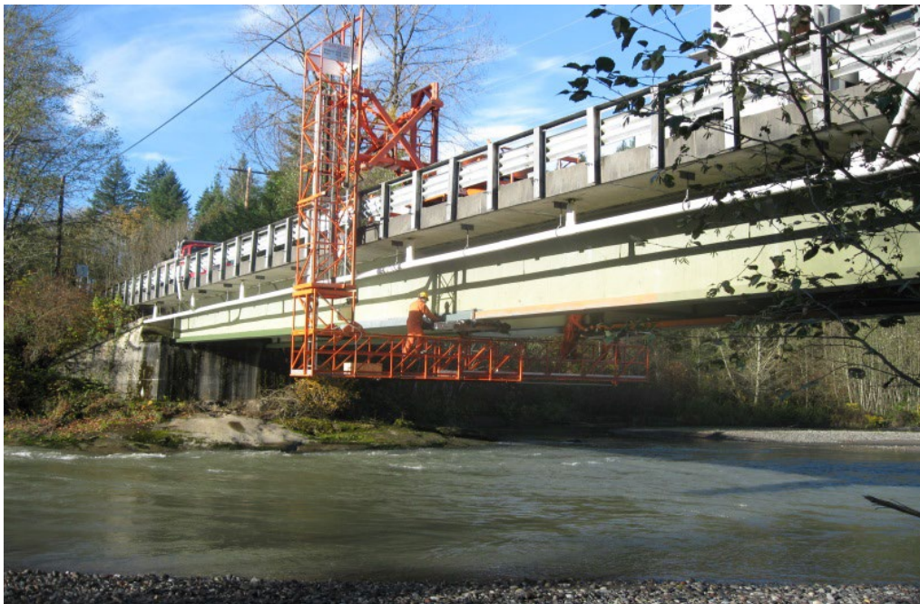
Photo of M&O's bridge inspection platform in use on Mosquito Lake Road/NF Nooksack River Bridge No. 332
