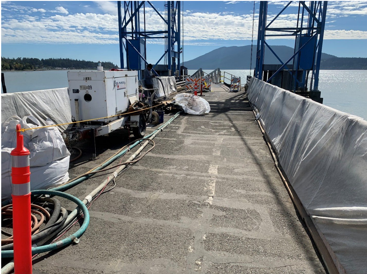
Picture of terminal preservation work at the Gooseberry Point ferry terminal.
