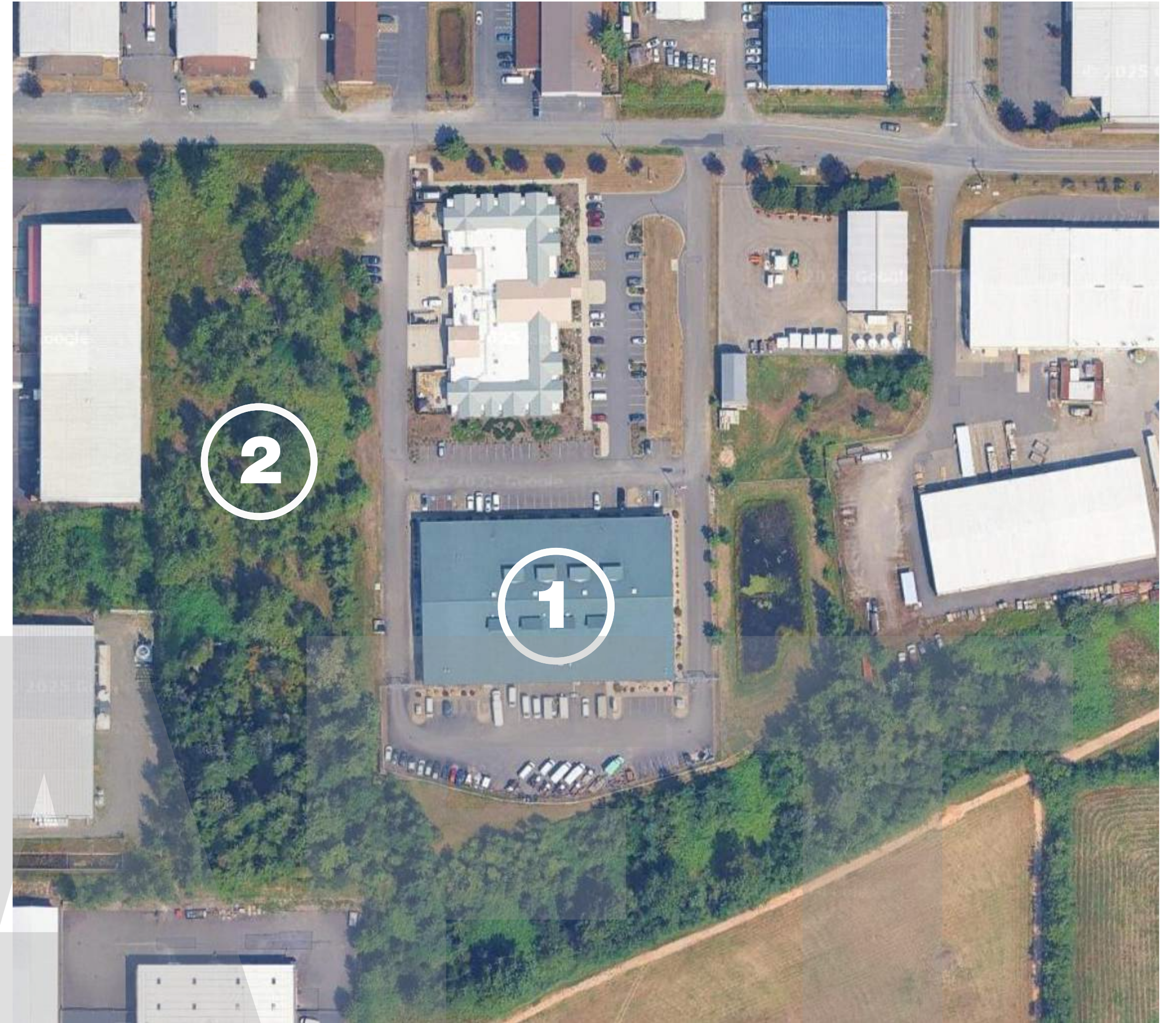
SITE 2: 2000 Division St.
