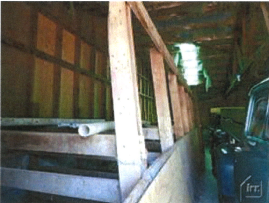
15. Interior of storage building
