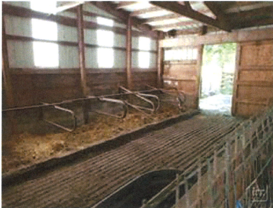
19. Interior of Barn 2
