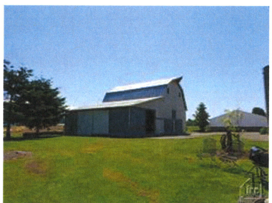
12. North and west sides of barn 1
