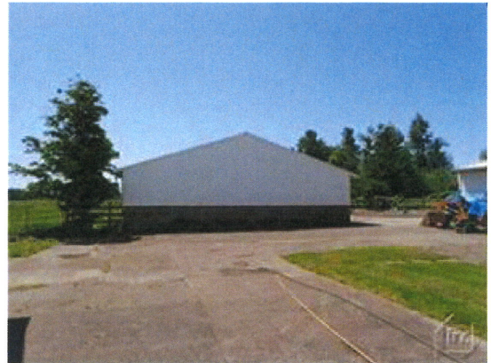
14. North side of storage building
