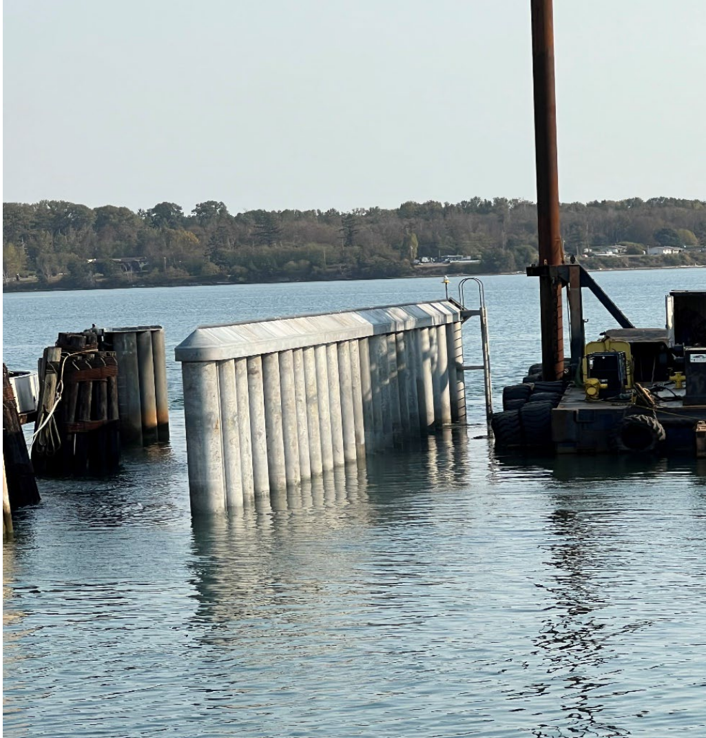
Picture of newly completed Lummi Island Breakwater at the Lummi Island ferry terminal.
