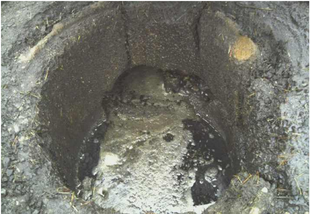
Figure 4-3. Catch Basin with Oil Sheen and Odors (photo by Wilson Engineering)
