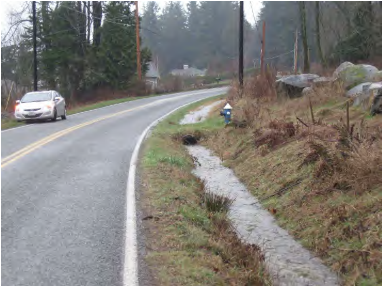
Figure 4-1. Roadside Ditches on Semiahmoo Drive, Undersized for Large Storms
