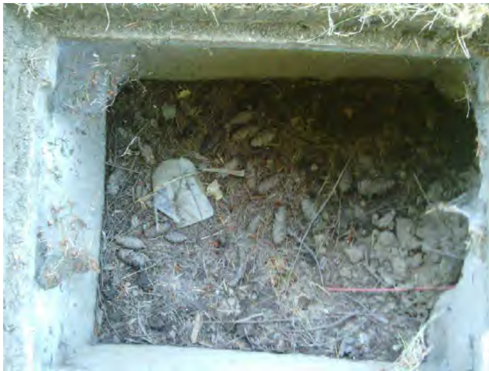
Figure 4-4. Catch Basin with Sediment and Debris Accumulation (photo by Wilson Engineering)
