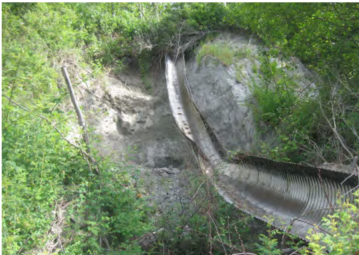
Figure 4-2. Erosion-Undermined Storm Drain Outfall to Birch Bay
