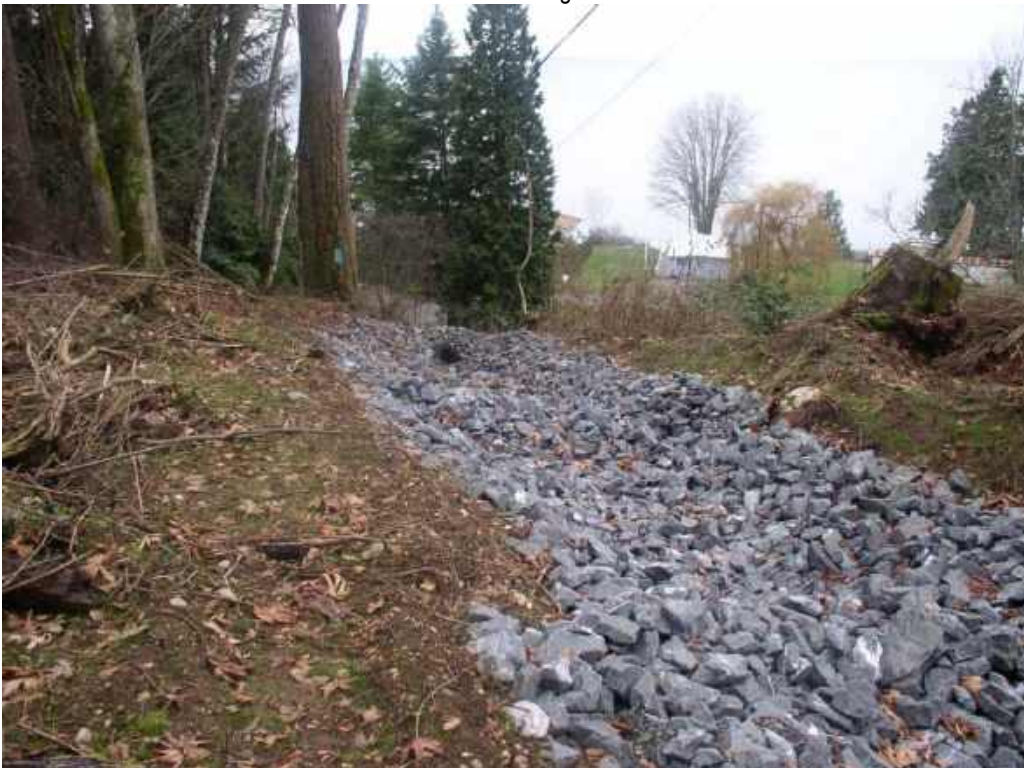
FIGURE 2 Modifications made to Channelized Stormwater Flow along Semiahmoo Drive in Birch Point Area
