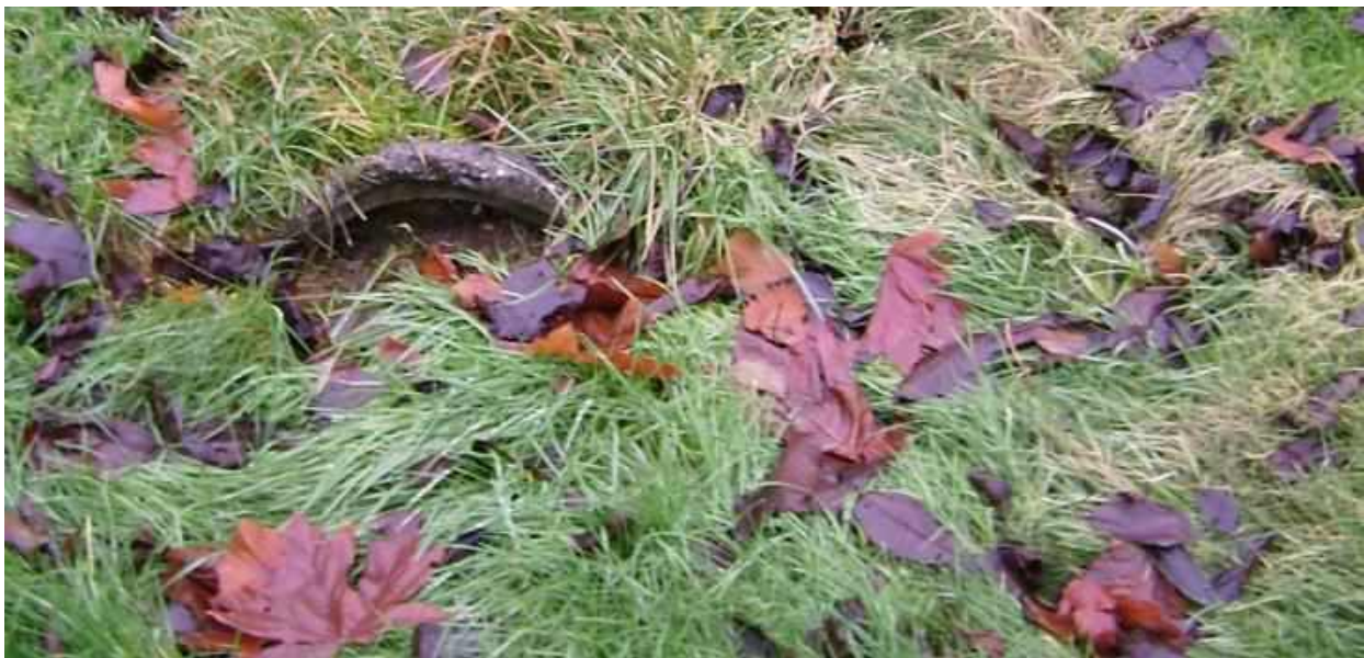
Figure 4-2. Blocked Culvert
