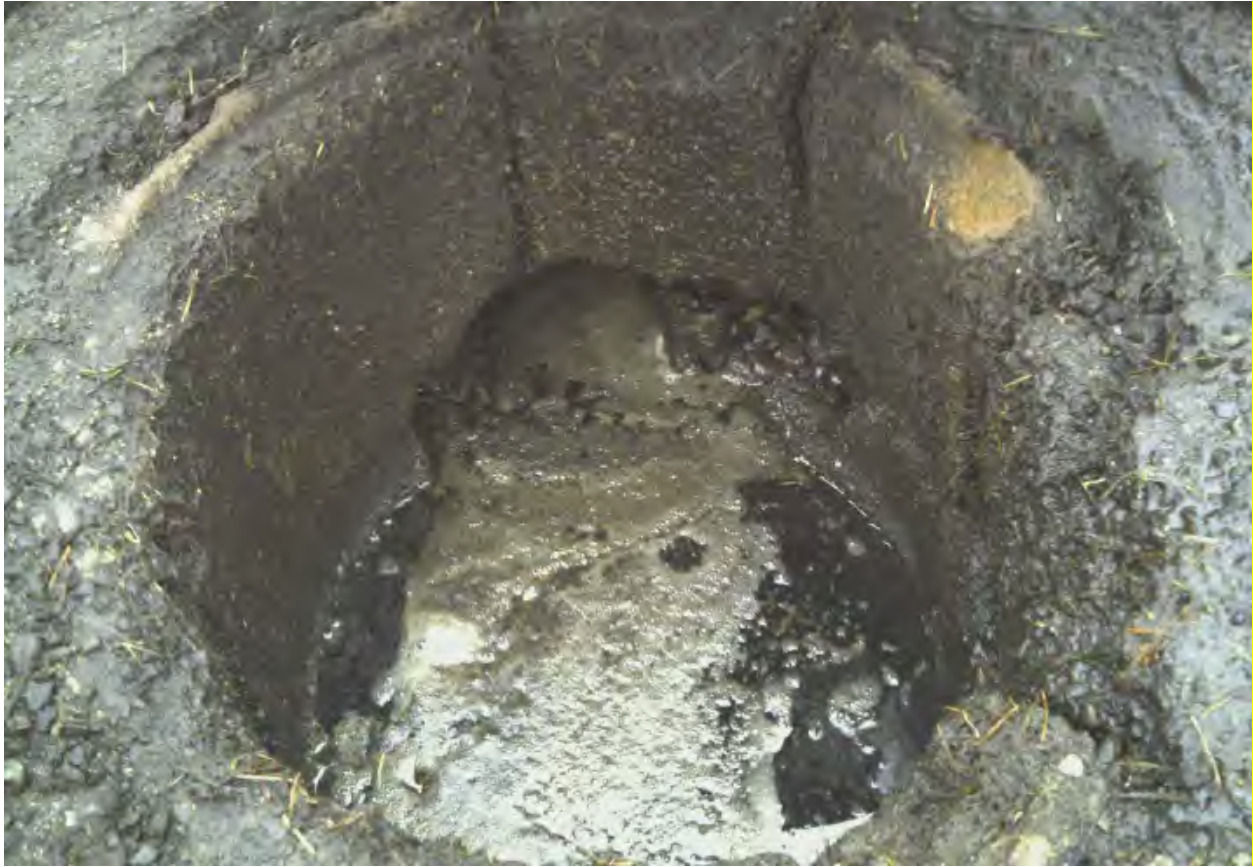
Figure 4-3. Catch Basin with Oil Sheen and Odors
