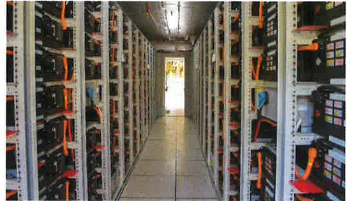
A view of the battery at the Glacier substation.
