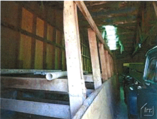
15. Interior of storage building
