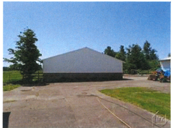
14. North side of storage building
