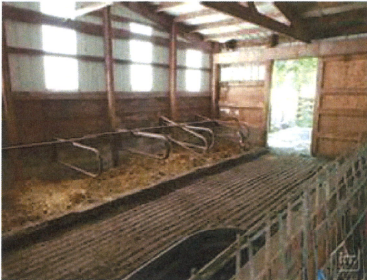
19. Interior of Barn 2
