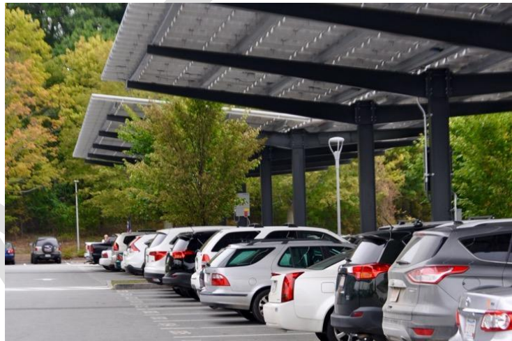
Figure 2.20. Dual-use parking lot and solar panels. Credit: Masha Yakhkind.
