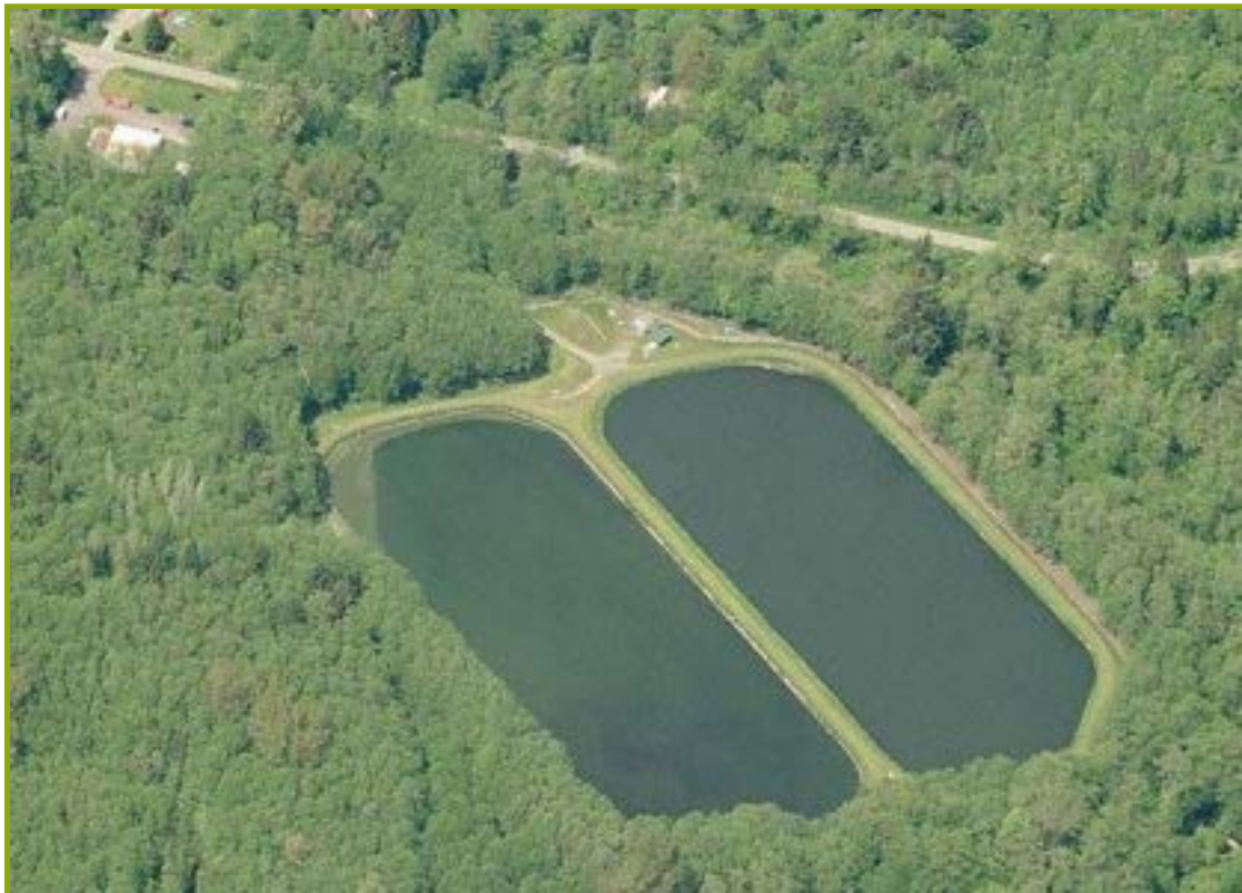
Figure 2.4 - Aerial View of Lake Samish Lagoon Treatment Facility
