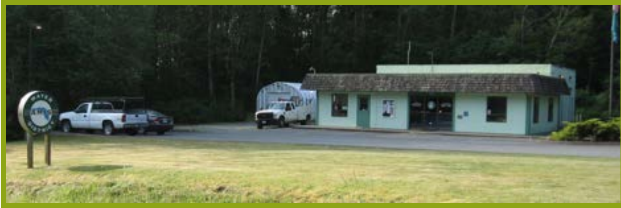
Figure 2.1 - Samish Water District Headquarters (2195 Nulle Rd., Bellingham, WA)
