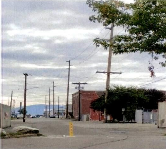
C Street looking westerly. The City will complete sewer and street infrastructure C Street from Bancroft to Holly Street. EDI funds would pay to underground overhead wires and add intersection streetlights.
