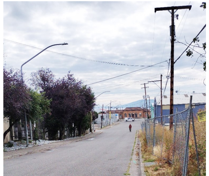
Figure 5. View looking westerly down D Street with the historic BNRR Depot at the terminus. EDI funding would remove utility poles and overhead wires.
