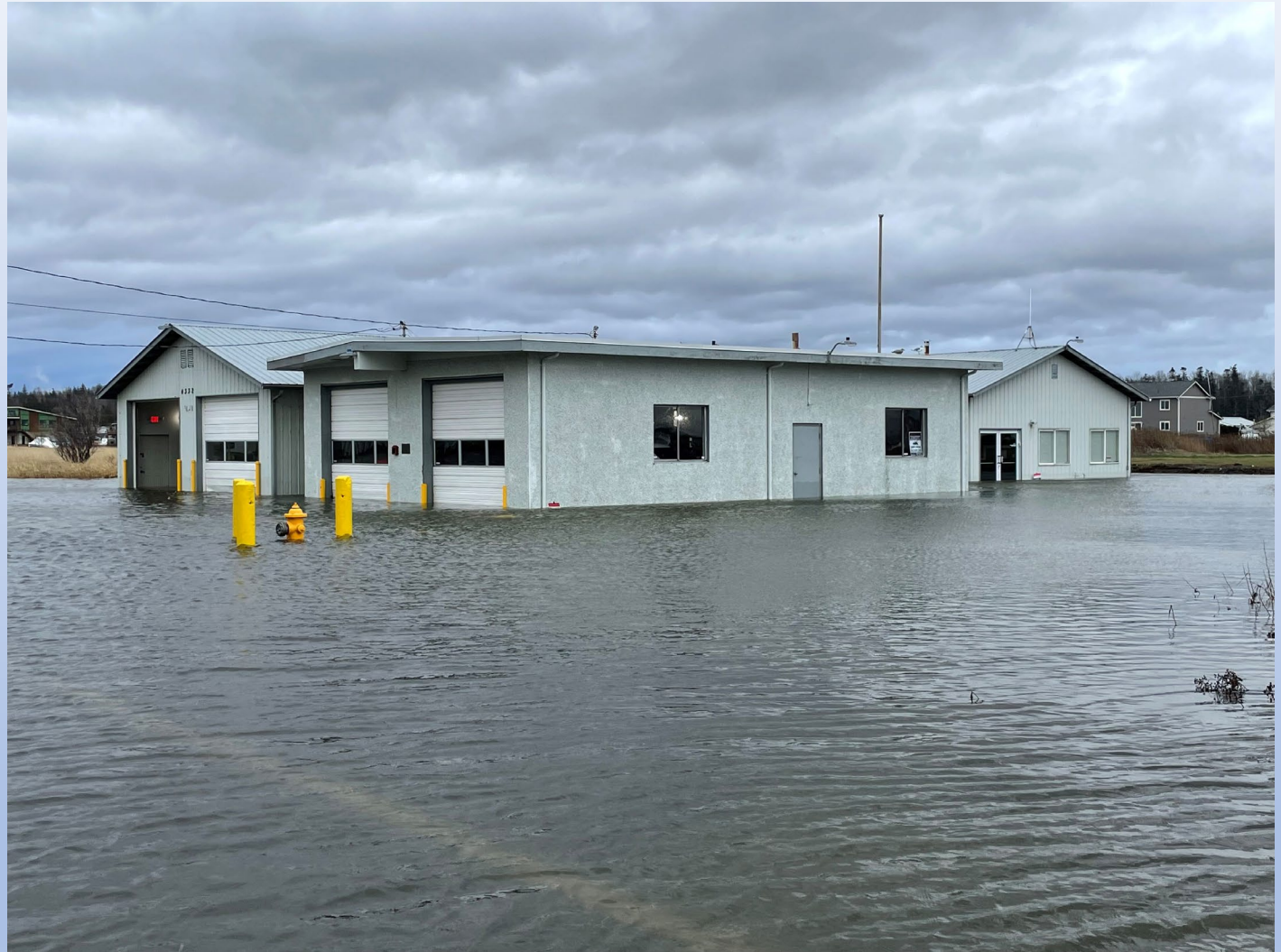
Photo: Exterior Whatcom County Fire District 17 Station, Sandy Point - King Tide Event 2022
