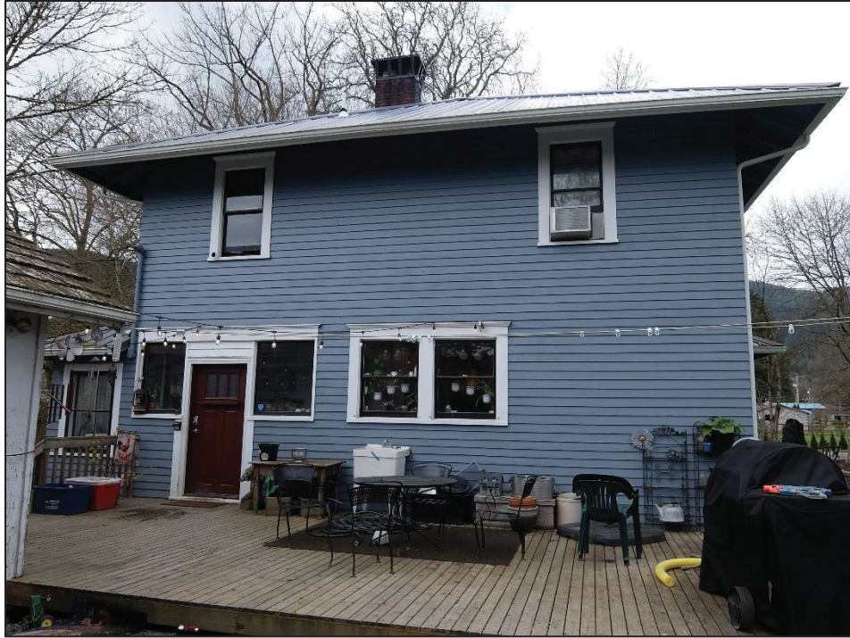
WESTERLY VIEW OF RESIDENCE
