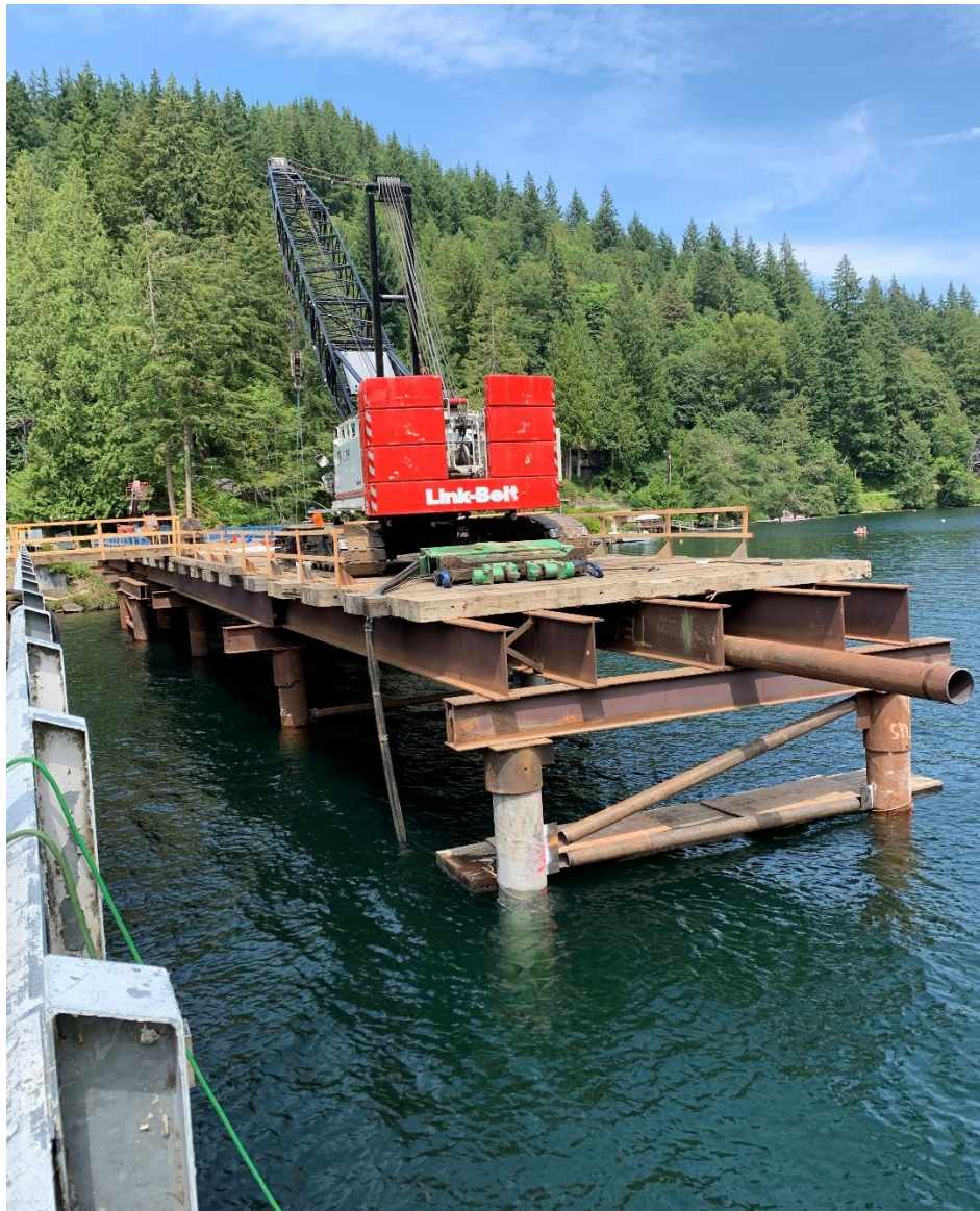
Temporary work bridge under construction on the North Lake Samish Drive Bridge No. 107 Replacement Project.
