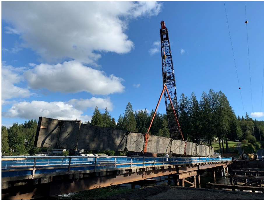
Demolition of old North Lake Samish Road Bridge No. 107.
