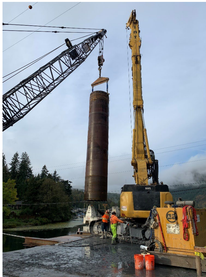
Installation of drilled shaft on the North Lake Samish Drive Bridge No. 107 Replacement Project.
