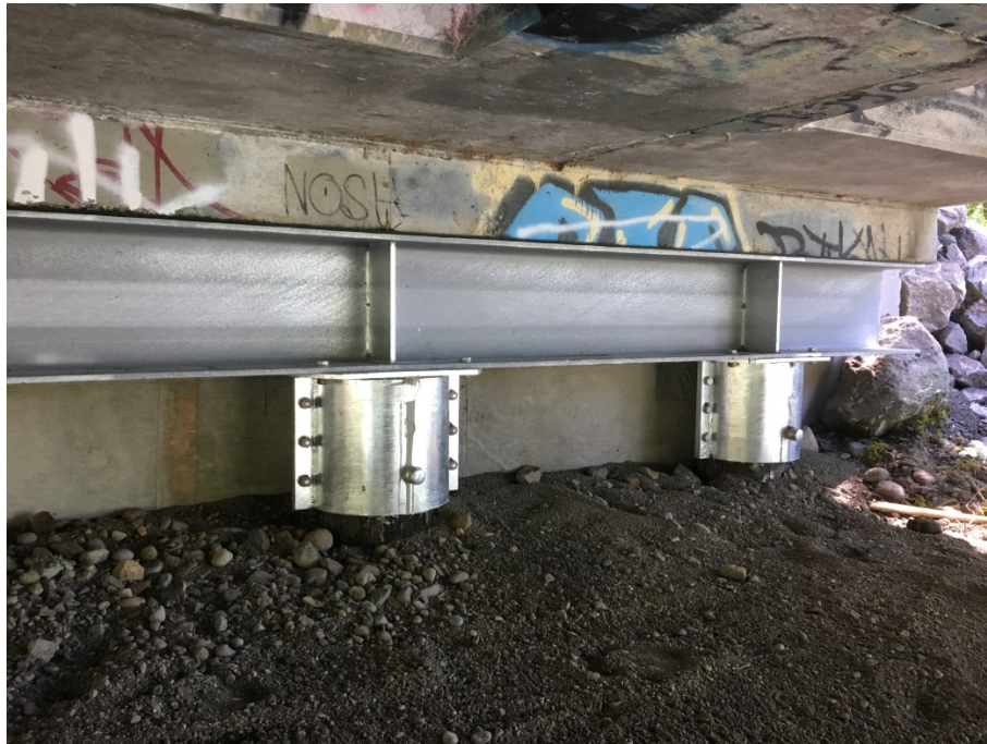
Photo of the new steel I-beam cap and steel pile collars
