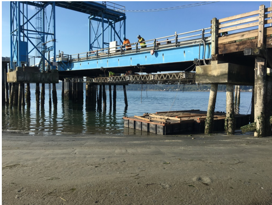
Gooseberry Point terminal structural steel repair work
