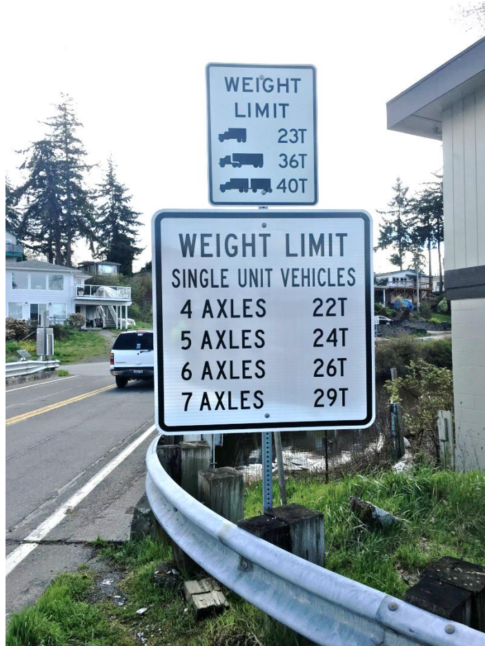
Posted weight restrictions for Jackson Road/Terrell Creek Bridge No. 81
