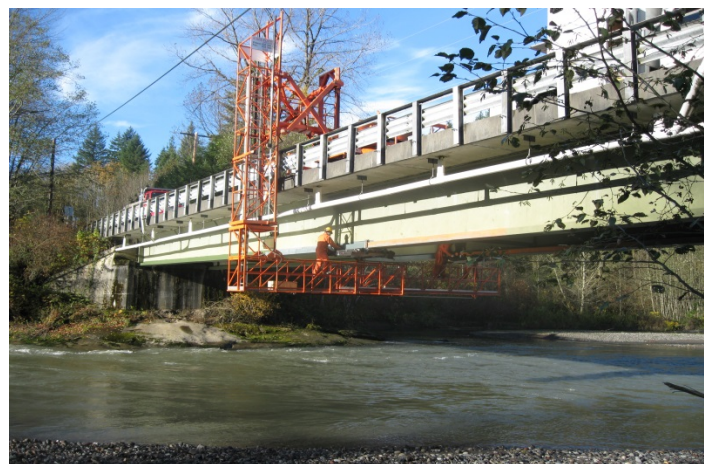
Maintenance & Operations crews deploying the hydra platform on Bridge No. 332
