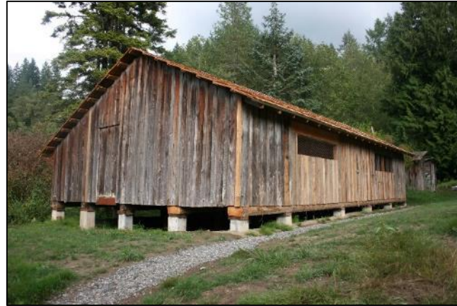
Nesset Farm Utility Barn
