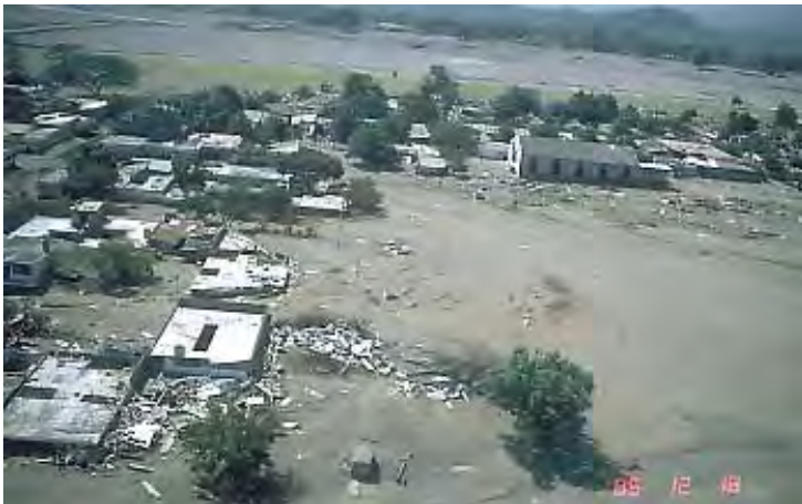
Photo of a lahar and damaged buildings.
