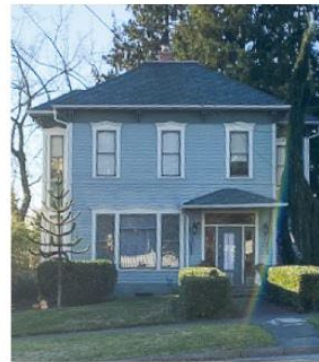
Duplex Stacked 2 units
