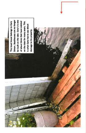
Note: Upper picture – This is the original picture in the Document. Wood is rotten and no longer structurally sound. This boat house has not been kept in good repair by the owner.
