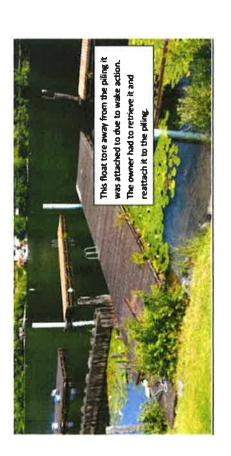
Note: Upper right picture – two separate floats are connected by wood that is severely decayed and is not structurally sound to bridge two floats. The float on the left side of the picture has top boards that are badly worn. Top boards on left dock have been replaced which is good. (photo taken from public waterway, July 27, 2019)
